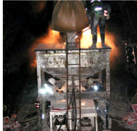
Figure 8. Cement Hooper and Pump Configuration.
