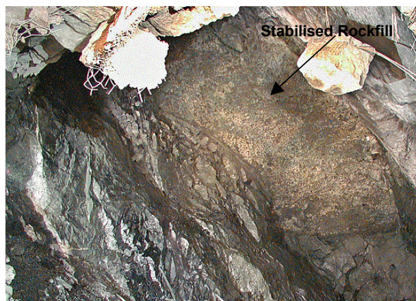
Figure 10: View from Beneath 955 Stabilised Rockfill Pillar.
