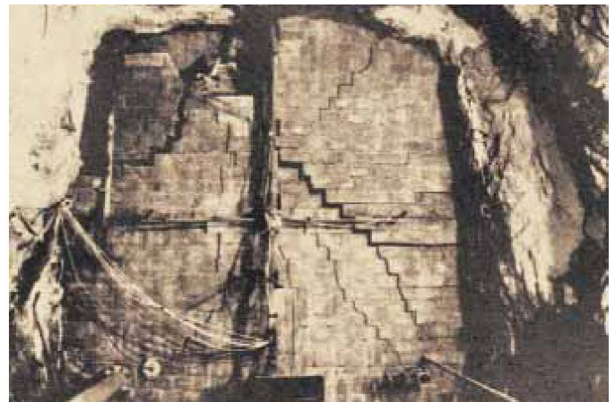
Fig. 4. Masonry bulkhead pressurized to 750 kPa at the Mt. Isa Mine (Grice, 1989)
