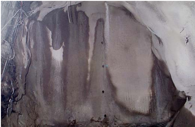
Fig. 1. Typical sprayed shotcrete/fibrecrete paste bulkhead.
