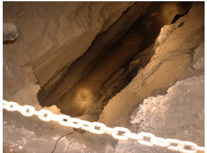
Fig. 8. Mine B stope ready to be filled.
